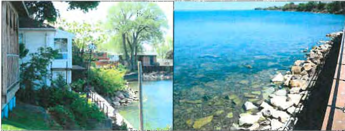
Shoreline Erosion Protection
