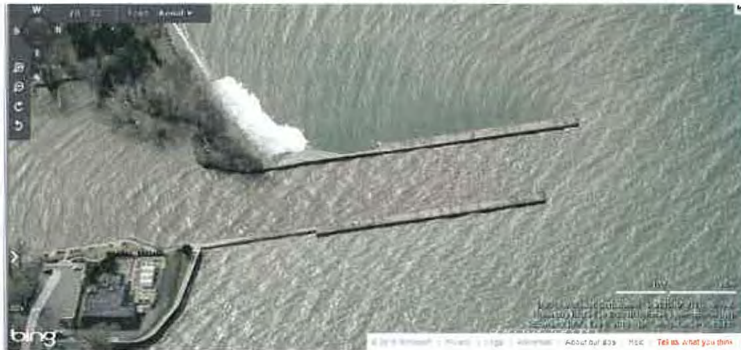
The Entrance Channel to Wilson Harbor and Tuscarora Bay
